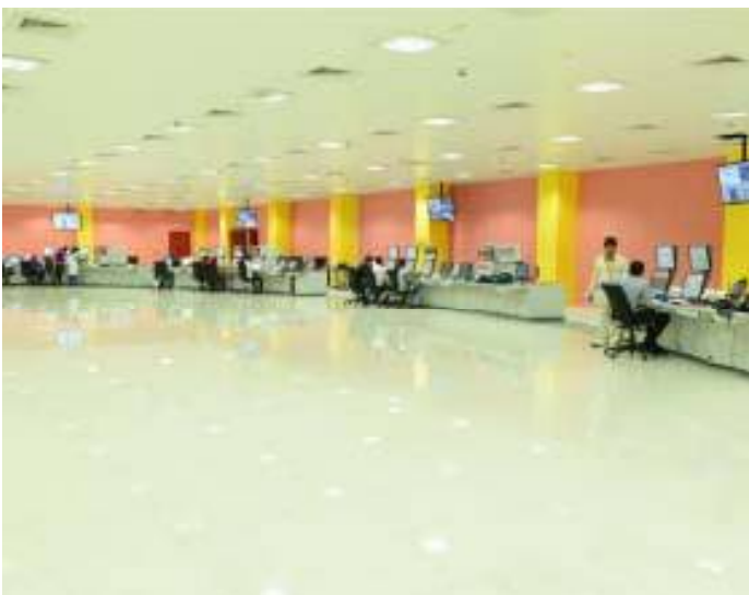
Master Control Room
