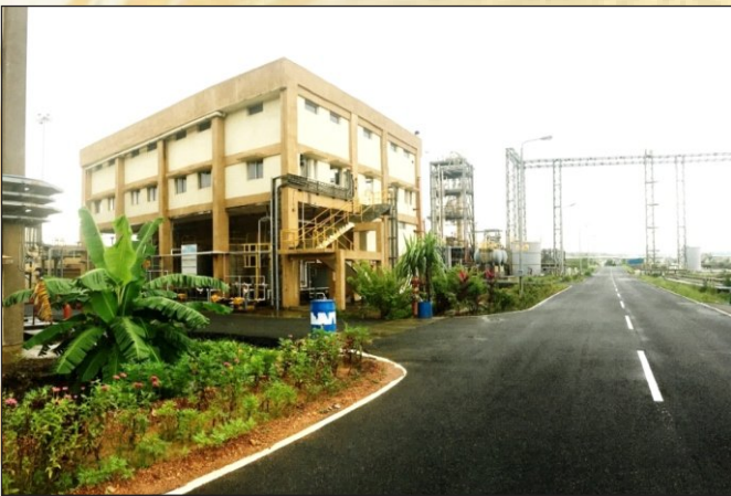
Electrical Substation inside Aromatic Complex
